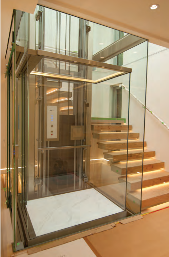
UT Elevator installed a cab with all four sides made of clear-glass panels with mitered glass edges within an all-glass hoistway without corner posts.
